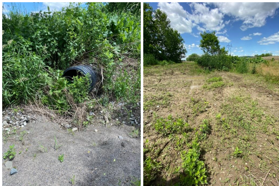
Figure 4: Left photo shows the existence of an outlet pipe from the stormwater feature located in Wetland AA. The right photo shows the discharge area from the stormwater outlet. While a concave area is present, the Corps determined the feature to be indiscrete primarily due to the lack of evidence of flow particularly since the area experienced recent heavy rains.
